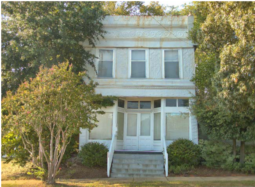
Toomer Building (extant) at 735 Carroll Street, Perry, Houston County, built in 1905. Brian Brown, 2023.
