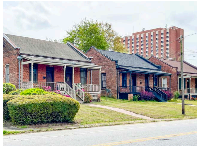
Double Pen Houses, Monroe Street in Macon Historic District (NRIS #74000658), Bibb County [extant]. Ethos Preservation .
