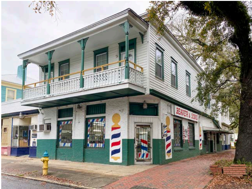
Beaver & Sons Barbers (extant) at 2515 Martin Luther King Jr. Blvd., a contributing resource to the Cuyler Brownville Historic District (NRIS # 98000028) Savannah, Chatham County. Ethos Preservation.
