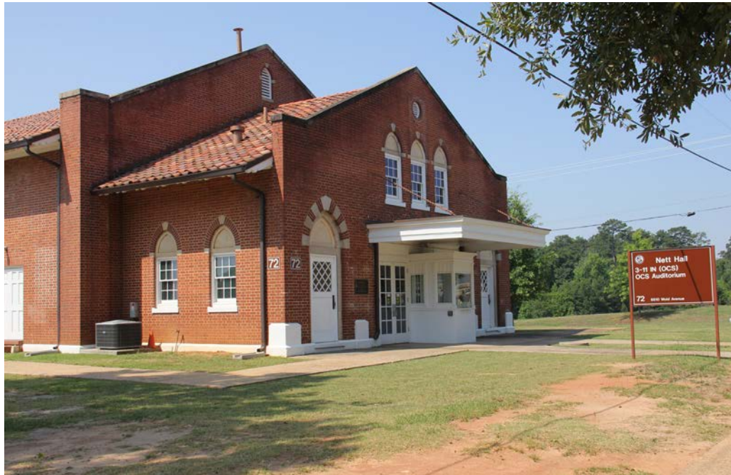
Nett Hall [extant], Fort Moore [formerly Fort Benning], Columbus, Muscogee County. U.S. Army photo by Edward Howard, U.S. Army Garrison Fort Benning Directorate of Public Works .
