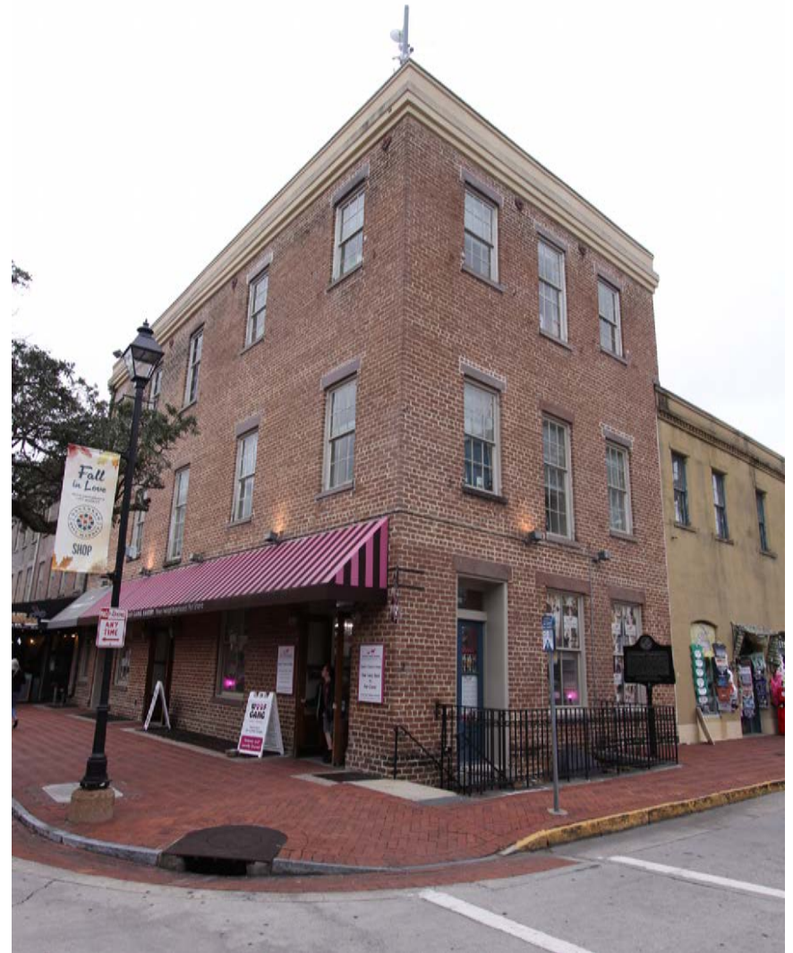
The Montmollin Warehouse at 2020 W. St. Julian Street, within the Savannah Landmark District (NRIS #66000277), Chatham County. Ethos Preservation.
