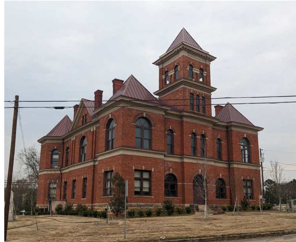
The Madison County Courthouse [extant] (NRIS #80001114) at 101 W. Courthouse Square, Danielsville, Madison County. Building was the site of multiple racially motivated trials including the trial of the men who murdered Lt. Col. Lemuel Penn. Ethos Preservation.
