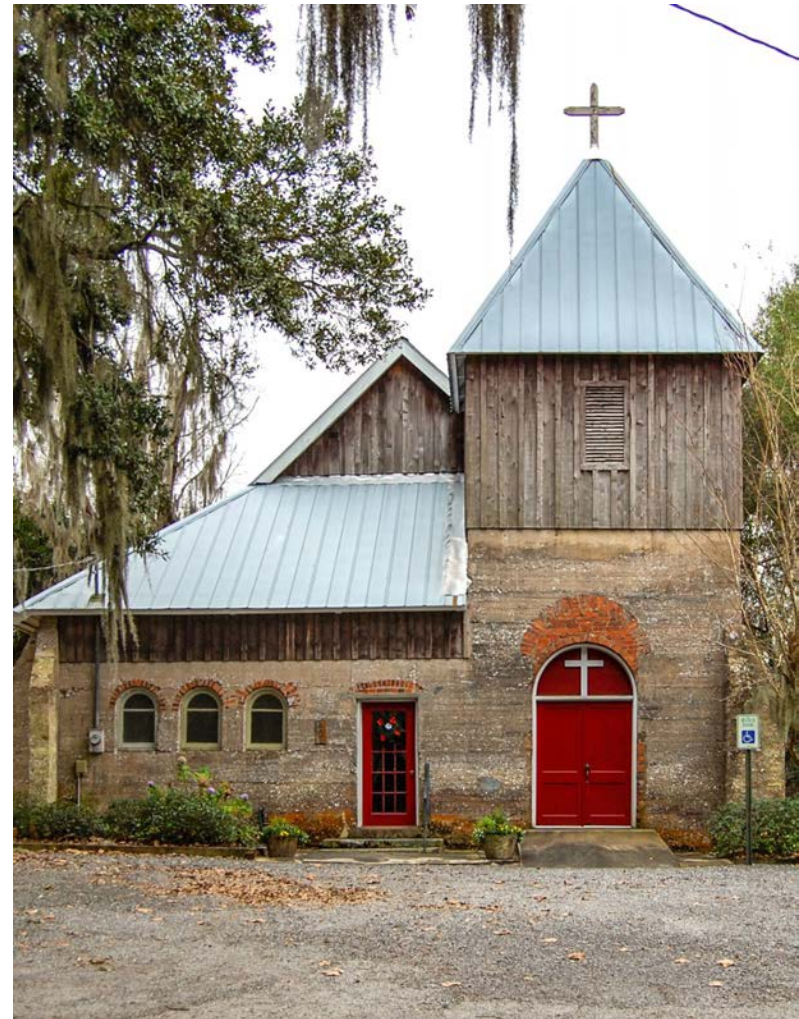
St. Cyprian's Church (extant) at 401 Fort King George Drive in Darien, McIntosh County, a contributing resource to the Vernon Square-Columbus Square Historic District (NRIS #85000581). Built c.1876 and constructed of tabby and still in use today. Rebecca Fenwick.
