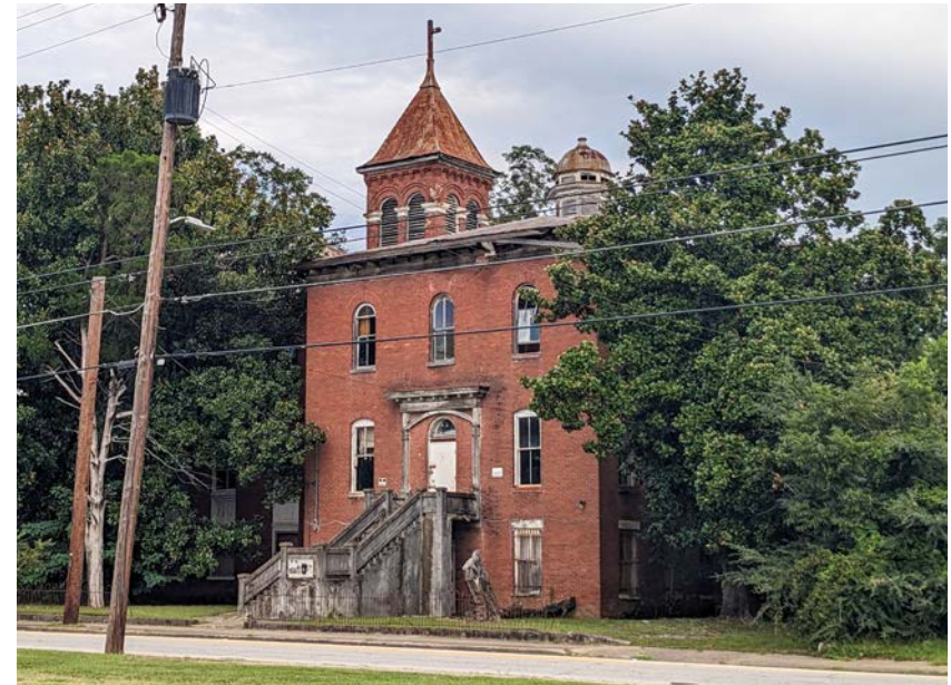
St. Benedict of the Moor Industrial School (extant), 12th Street south of Laney Walker Blvd. in Laney Walker North Historic District (NRIS # 85001976) in Augusta, Richmond County. Ethos Preservation .
