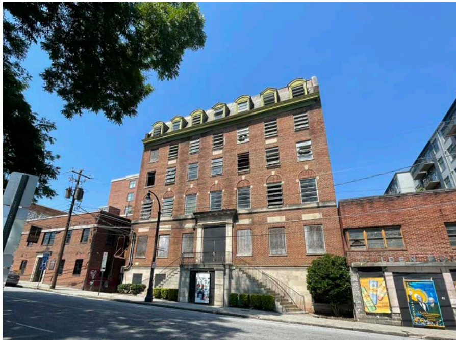
Butler Street YMCA (extant), 22 Jesse Hill Jr. Drive NE, Atlanta, Fulton County, a contributing resource to the Sweet Auburn Historic District (NRIS #76000631). Danielle Meunier.
