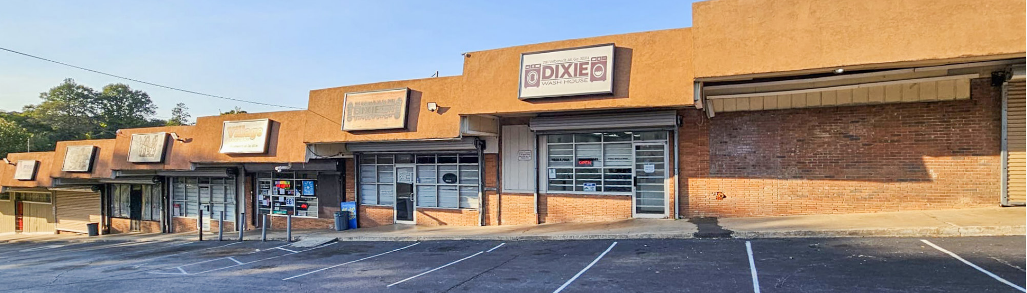
Dixie Hill Shopping Center at 2179 Verbena Street, Atlanta, Fulton County. Timothy Deptula.
