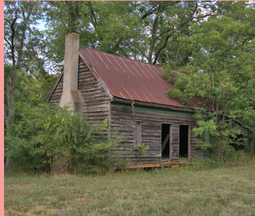
Boswell Tenant Housing at 1464 US-129, Eatonton, Putnam County. Built in the early 1800s as a Double-Pen with a side gable roof. A small family cemetery also exists on the lot. This resource is included in the National Register Nomination as an outbuilding to the Historic Tompkins Inn (NRIS #78001002). Brian Brown, 2022 .
