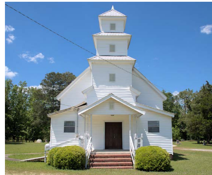
Central Tower Church, Black Rock A.M.E. Church at 441 S. Hulin Avenue, Tignall, Wilkes County (extant). Brian Brown.
