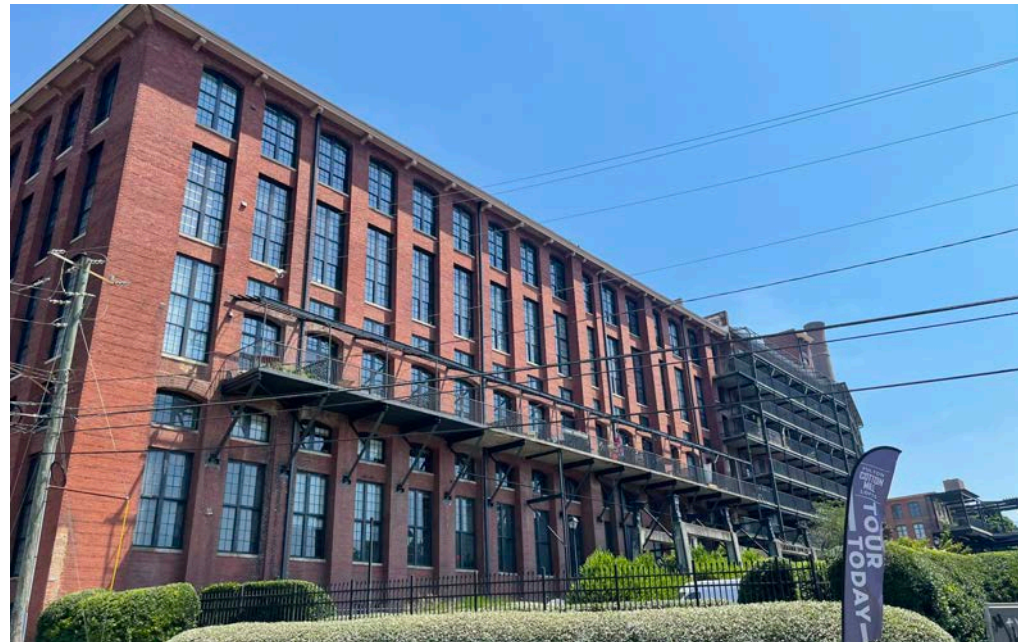
Fulton Bag and Cotton Company (extant) a contributing resource to the Cabbagetown Historic District (NRIS #76000623) at 170 Boulevard Avenue, Atlanta, Fulton County. Danielle Meunier .
