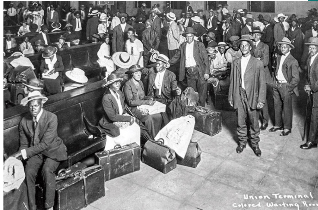
Train Station Waiting Room, Headed North. Eastern Connecticut State University.
